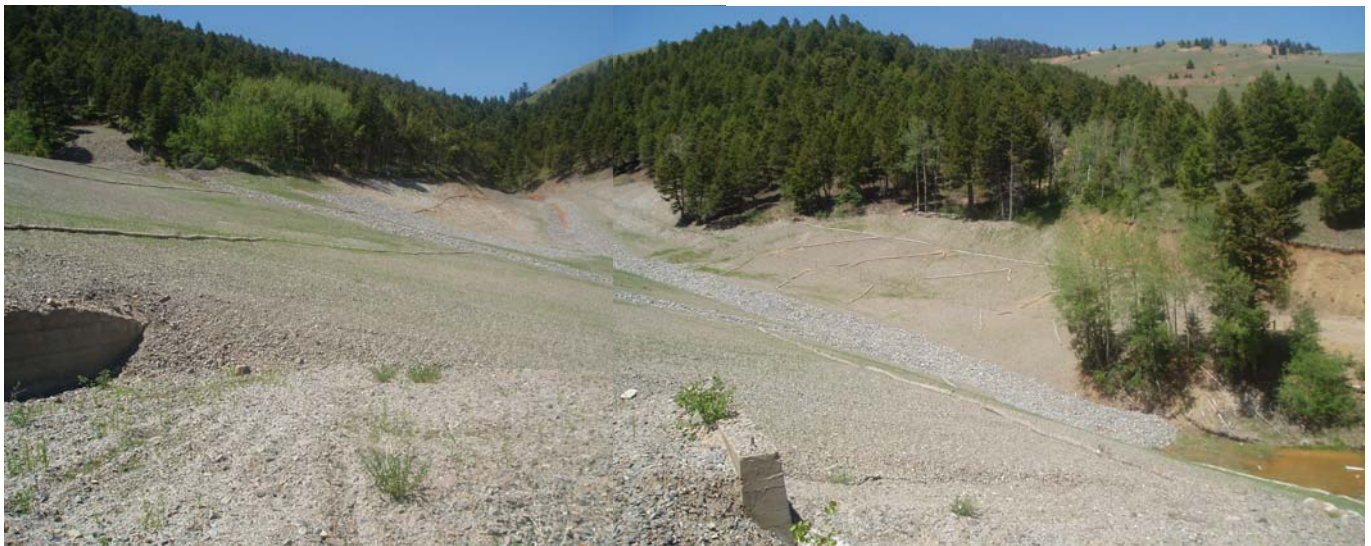
Washington Mine & Mill , photos above June 2007 (during reclamation) & below June 2008 (reclamation complete) showing mill foundation, mine & mill wastes and hazardous equipment and facilities removed, stream channel reconstructed, high altitude revegetation
