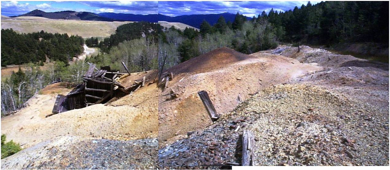
Washington Mine & Mill , photos above August 2005 (before reclamation) showing piles of mine & mill wastes and hazardous equipment and facilities
