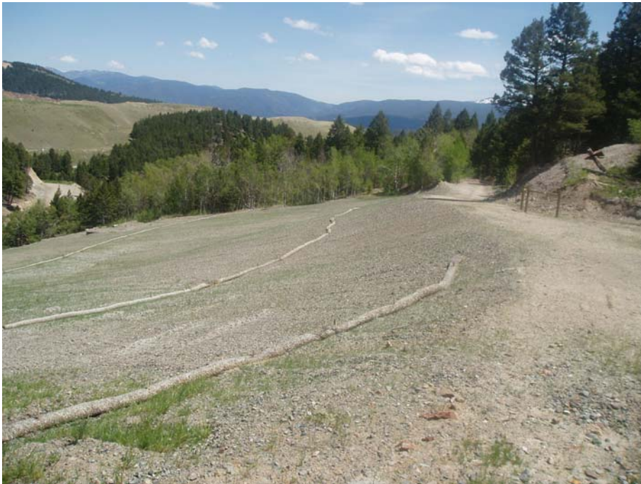
Washington Mine & Mill , photo left June 2008 (reclamation complete) piles of mine & mill wastes and hazardous equipment and facilities removed, high altitude revegetation
