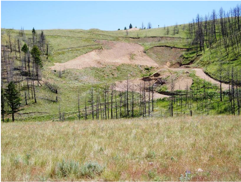
Belle Lode Mine , photo June 2007 (during reclamation) showing removal of mine wastes
