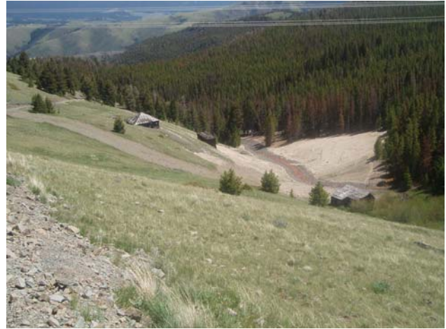
Bluebird Mine & Mill photos above & below June 2008 (reclamation complete) showing slight trace of acid mine drainage at head of channel, mine wastes piles removed
